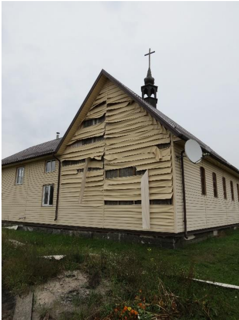
Signs of blast wave damage at St. Peter's Church, Makariv (Kyiv region). Photo by Ruslan Khalikov, September 17, 2022.
