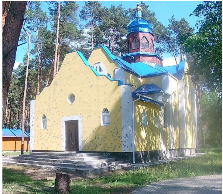
Shrapnel-damaged Church of the Intercession, Irpin (Kyiv region). Photo by Lyubov Kilikevska, May 28, 2022.
