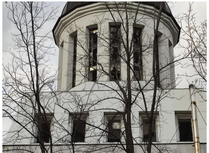
Windows blown out by the blast wave at St. Nicholas Church in memory of the victims of Chornobyl, Kyiv. Photo by Anton Leshchynskyi, March 22, 2024.
